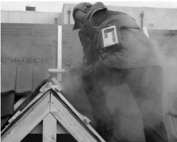
Figure 4 Sawing roof tiles
