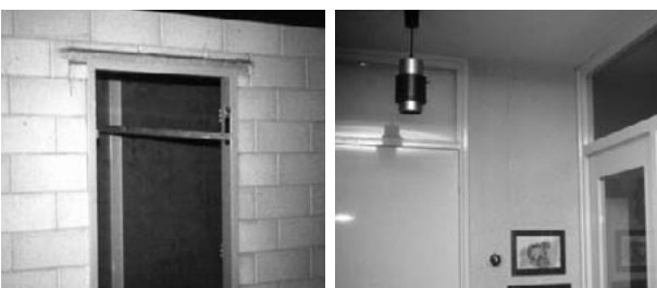
Figure 13 Door opening with a lintel
