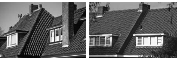
Figure 5 Valley gutter and angle ridge construction
