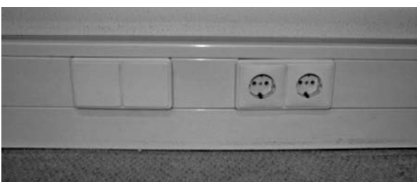
Figure 20 Cable gutter
