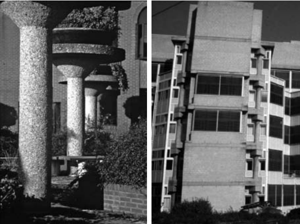
Figure 2 Grit blasted columns
